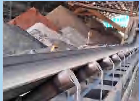
Fig – LINEAR STACK RECLAIMER
